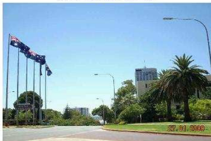
LED Street Light, LU6 in Australia
