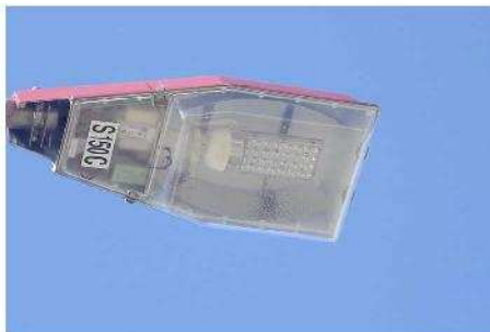
LED Street Light SP90 in New Zealand
